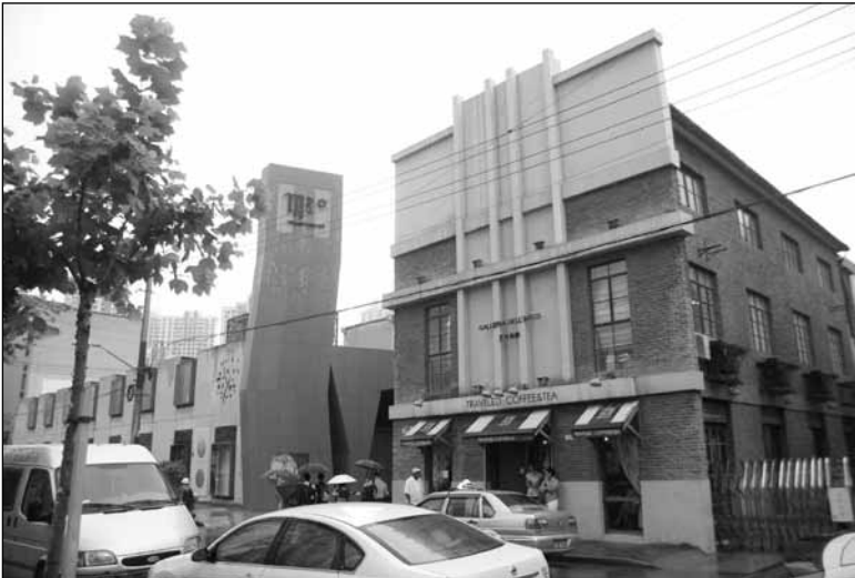
Fig. 2. Renewal of post-industrial space for “Creative Garden”, Shanghai. Source: photo by D. Wiśniewska.
